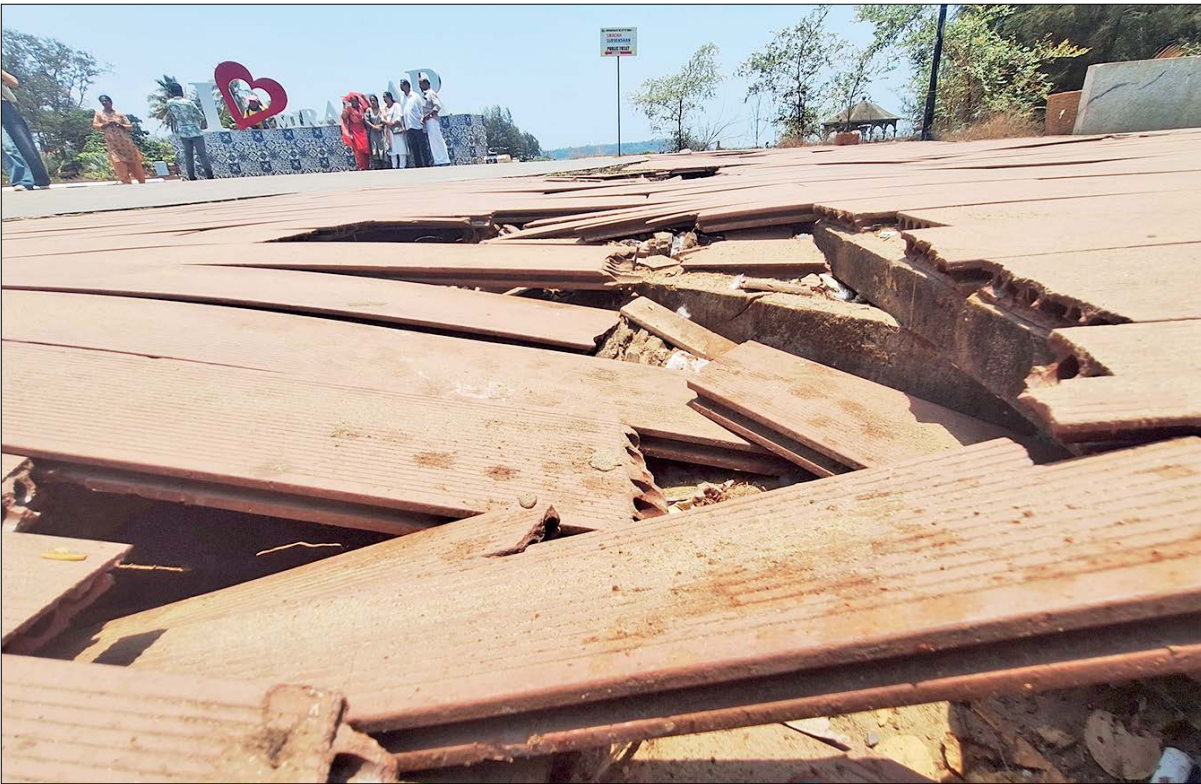
Broken pavement tiles at Miramar promenade pose safety risks to beachgoers, blamed on vehicular movement along the beachfront
