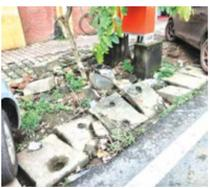
Square to the IOC Terminus. The problem began after the pavements were dug up for laying underground cables. Citizens had hoped the walkways would be restored with new pavers once the work was completed—but that never happened. Now, with the onset of the monsoon, the condition has only worsened.
