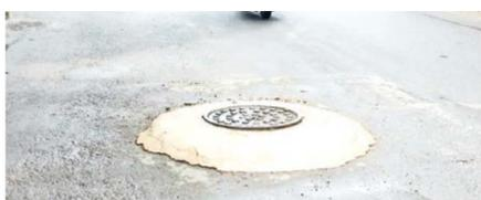
and the raised manholes become hard to spot. In an attempt to avoid them, riders may swerve into the path of oncoming traffic, increasing the risk of head-on collisions and accidents. Ideally, the manhole covers should have been installed flush with the road surface along the entire stretch. Now, the only
