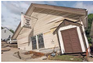
The Valley Grove Assembly of God, twisted and moved from its foundation by floodwaters, in Valley Grove, West Virginia
