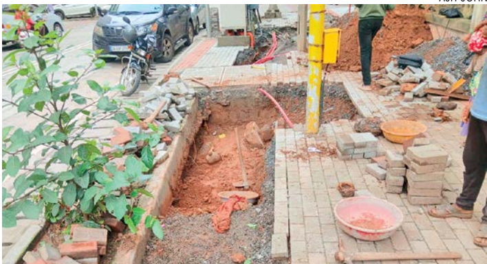
Pavers of the footpath at Tonca have been removed to install cables
