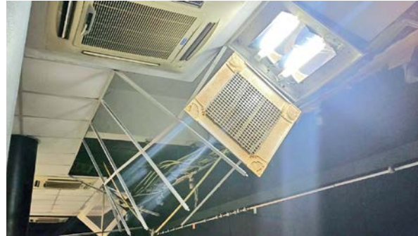
A section of the false ceiling which collapsed at the Ravindra Bhavan, Margao
