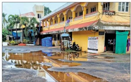
The recently tarred area around the Benaulim Panchayat Ghar has collapsed after the first spell of rain. The entire surface has sunk and
