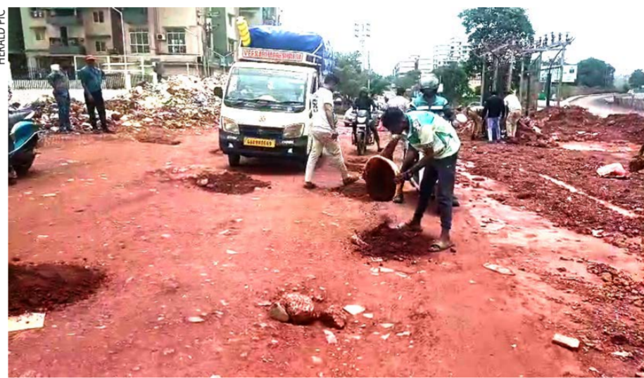
Potholed stretch near Umiya Building, Sancoale, being filled with stones and mud.
