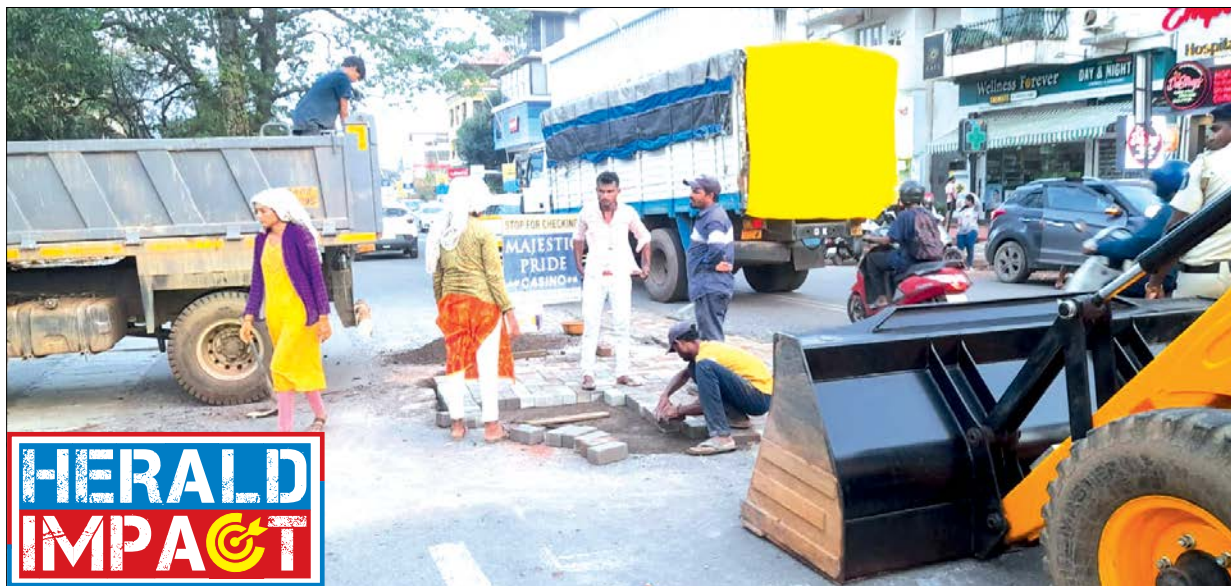
After O Herald published a photograph of potholes on the Chogm Road on May 26, authorities began repair work by placing pavers on the damaged stretch
