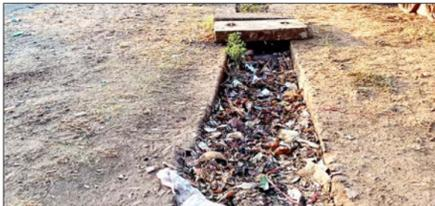
The drainage system around the market area in Chandor-Cavorim is in a deplorable state. Most drains are fully clogged with mud, plastic bags, bottles, palm fronds, and even broken concrete slabs. With the monsoon fast approaching, the risk of flooding is very real, yet the village panchayat seems to be turning a blind eye.
