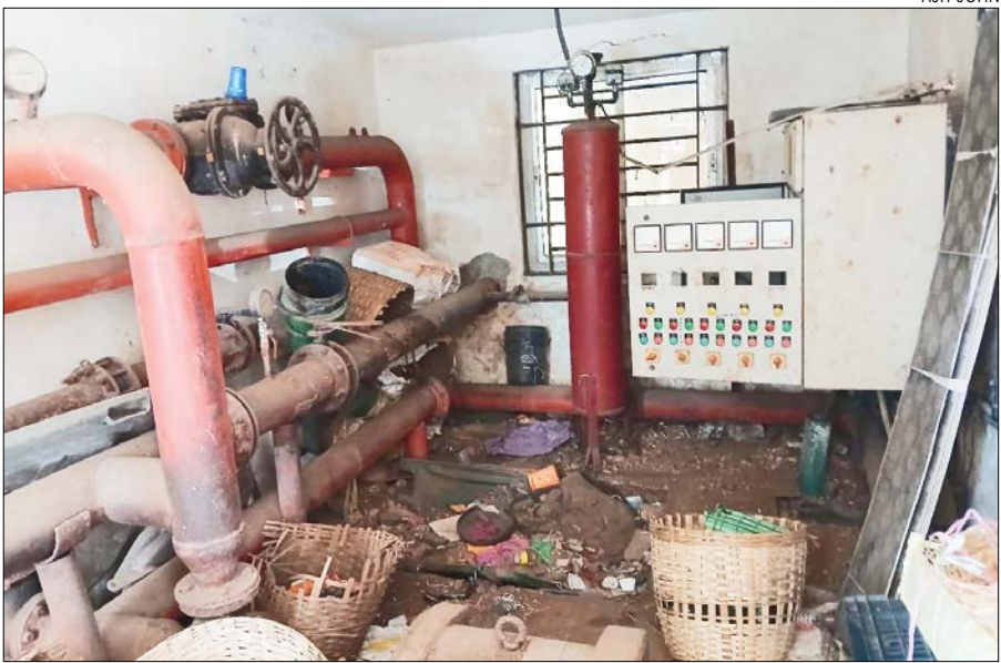
The fire hydrant station in an utter state of neglect
