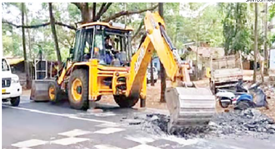
An earthmover removing the speed breakers
