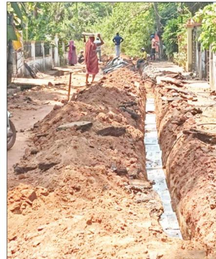
not only along either side but also across the middle at short intervals to accommodate the heavy-duty cables. Once the cables are laid, the potholes and trenches are not being properly filled, leaving large gaps and uneven surfaces. This has resulted in severe inconvenience for vehicles and motorcyclists, often causing damage to vehicles and even health issues like spondylitis among regular riders.
