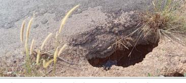
cember 17, with a request for the reconstruction of this precarious section of the road. Despite these notifications, the relevant authorities have seemingly not prioritized the complete rebuilding of the culvert. The application of temporary hot mix patches appears to be a superficial measure that has proven ineffective, as these repairs deteriorate repeatedly. It is unclear why a more permanent solution has not been implemented to ensure the safety of Goan citizens.
