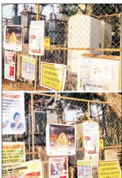
combustible materials would very likely lead to a fire. Given that these units are frequently located near buildings and power or internet cables, such an event could result in extensive damage and disruption.
