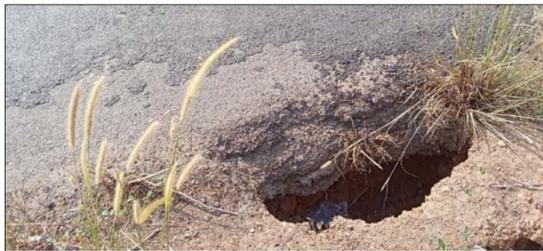
ember 17, with a request for the reconstruction of this precarious section of the road. Despite these notifications, the relevant authorities have seemingly not prioritized the complete rebuilding of the culvert. The application of temporary hot mix patches appears to be a superficial measure that has proven ineffective, as these repairs deteriorate repeatedly. It is unclear why a more permanent solution has not been implemented to ensure the safety of Goan citizens.
