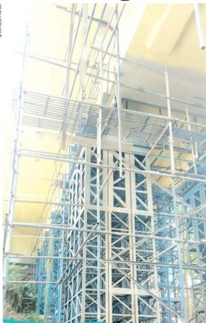
Major repair works were undertaken, including the addition of truss supports beneath the Borim Bridge
