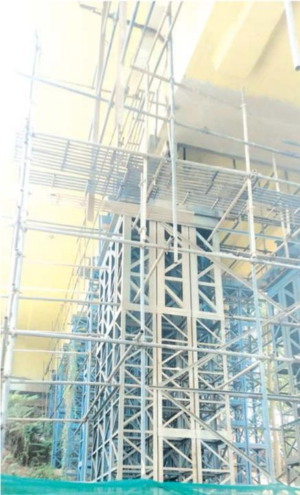
Major repair works were undertaken, including the addition of truss supports beneath the Borim Bridge
