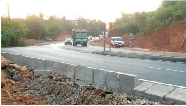
been progressing in the Ponda-Farmagudi area for the past year. However, following the widening of the road, the slope now appears to form a near right-angle, creating a hazardous curve due to the terrain's natural formation.
