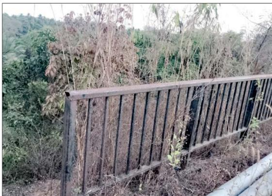
The Telaulim to Varca bridge in Salcete serves as a vital link for commuters, yet its railings appear to have been neglected, possibly since the time of construction. Several sections have fallen, as seen in the accompanying photograph. In the event of an accident, a victim could plunge directly into the River Sal, making urgent repairs and maintenance critical. The railings must be properly maintained to prevent further corrosion and ensure public safety. Additionally, it is important to
