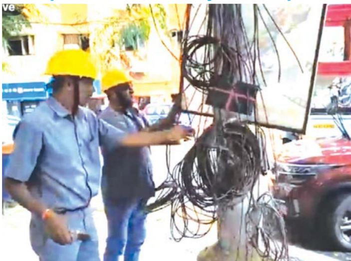
Linemen cutting the Internet cables installed on an electricity pole in the 18th June Road, in City
