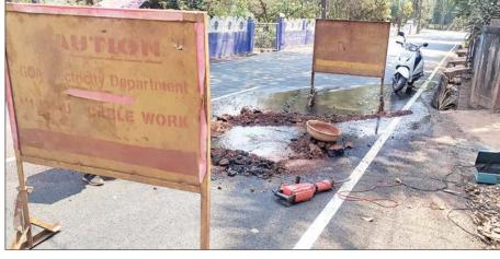
How is the cable handled and pulled through the conduit to its target? The hole drilling machine may save on excavations, but if such faults are going to occur in the future once the real load is applied to the cable, the hot spots will definitely lead to short circuits or open circuits. Consumers will suffer until the Electricity Department, with its new gadget, is able to locate the damaged spots—only time will tell.
