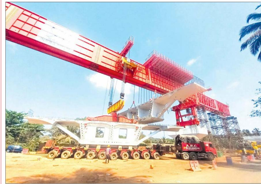
Gigantic cranes and other machinery are used to carefully position concrete box girders at the construction site of the elevated expressway near Guirim on Wednesday
