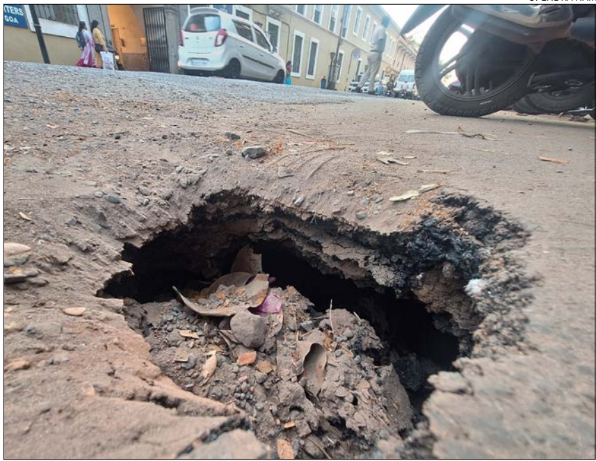
A small portion of the road in front of the Police Headquarters in Panjim has caved in, posing a hazard to pedestrians and passing vehicles
