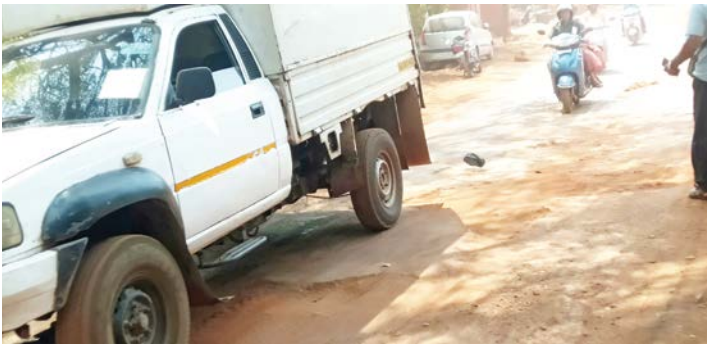
Motorists ply along the pothole-ridden stretch from Curti to Priol which was dug twice for laying underground electricity cables last year. The road is yet to be restored to its original condition
