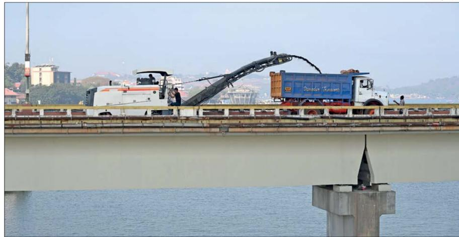
A road milling machine, also known as a cold planer, pressed into service on the Old Mandovi Bridge to remove asphalt. The bridge is expected to be closed for 15 days.
