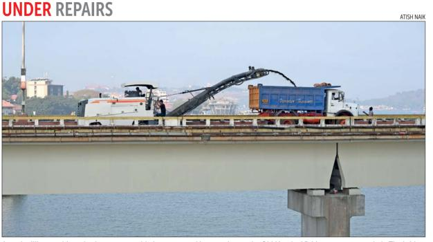
A road milling machine, also known as a cold planer, pressed into service on the Old Mandovi Bridge to remove asphalt. The bridge is expected to be closed for 15 days.
