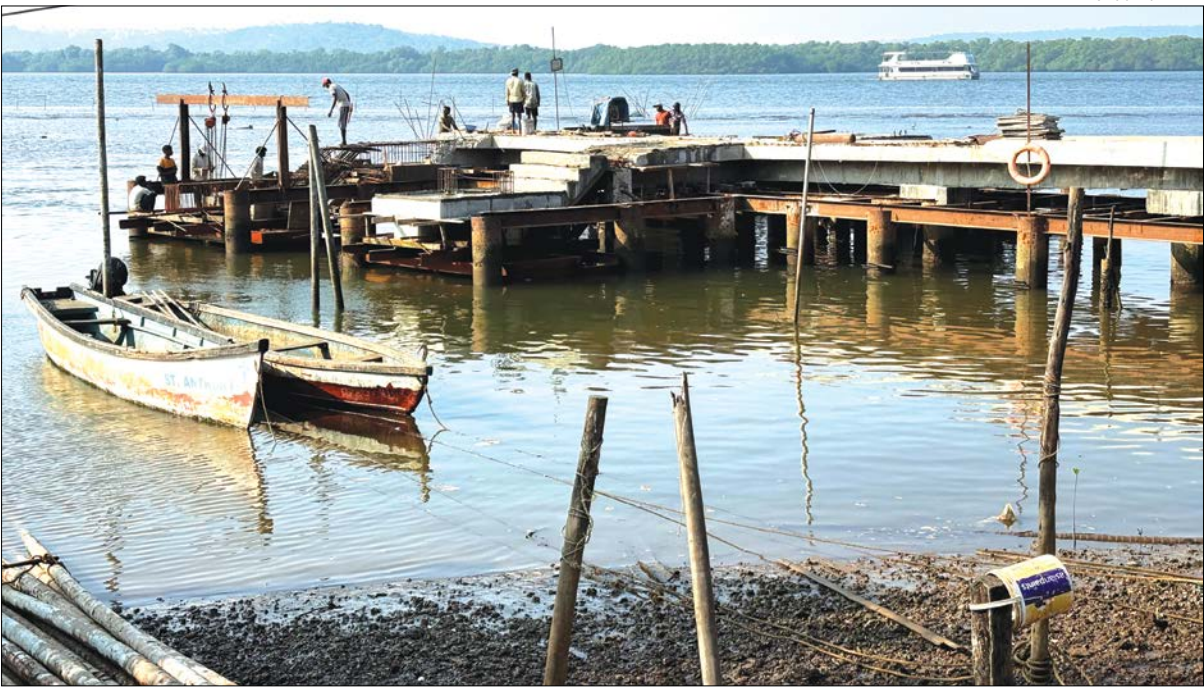
Labourers place concrete slabs on the jetty at Ribandar, which is being built under the Amrut Mission
