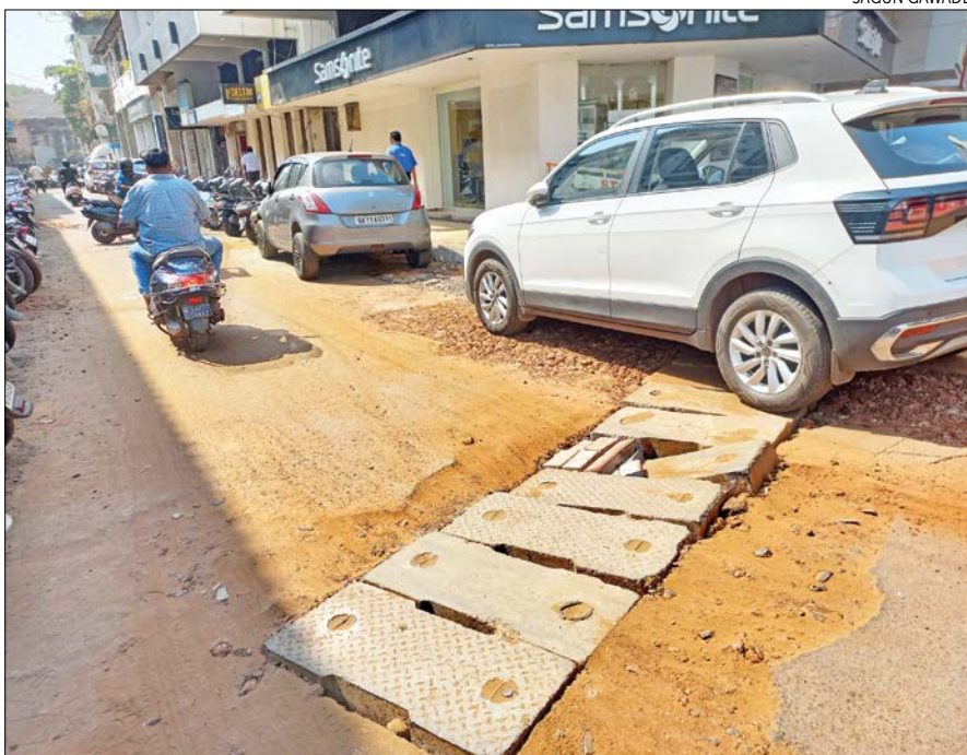
The authorities concerned have thought of a novel way of fixing things as the broken concrete slabs have been stuffed with pavers on the M G Road in Panjim
