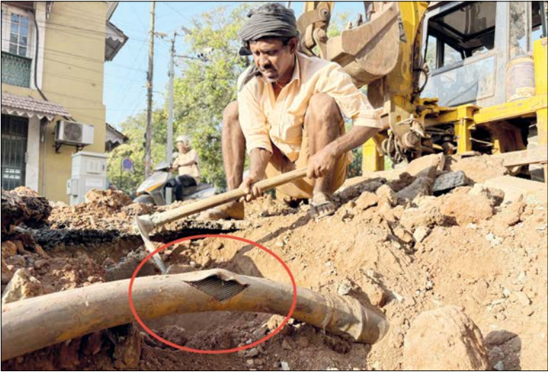
Barefoot and oblivious to the danger, a worker digs around a frayed electricity cable near Azad Maidan
