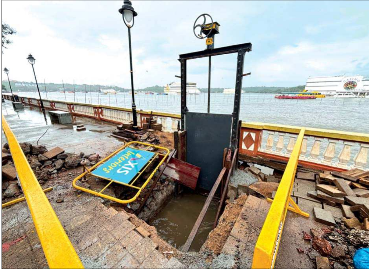
The water resources department and the Corporation of the City of Panaji (CCP) has installed a sluice gate along the promenade to mitigate flooding in Panaji during the monsoon opposite the ferry wharf
